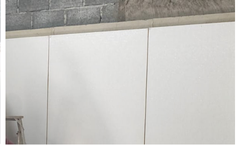
Glasbord® with Surfaseal® Sandwich Panels (Hygispan®)
